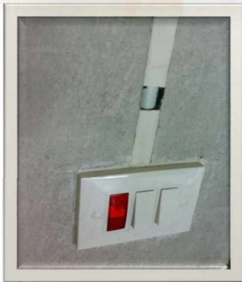
Concealed wiring & Switch Box
